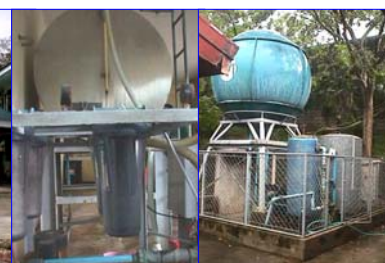
Water Filtration/ UV Light Treatment & Storage
